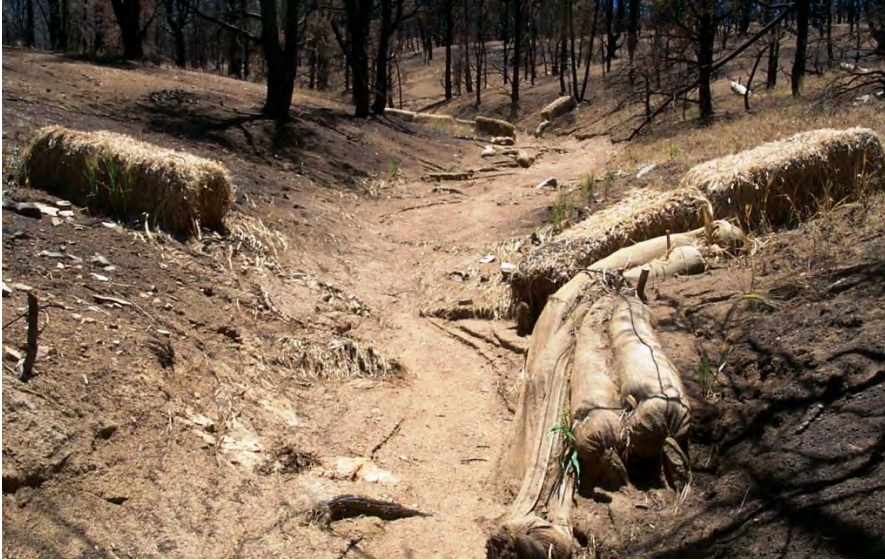
Figure 2: Failure of check dams with strawbales and wattles following an extreme rain event. Photo by Jan Beyers.
